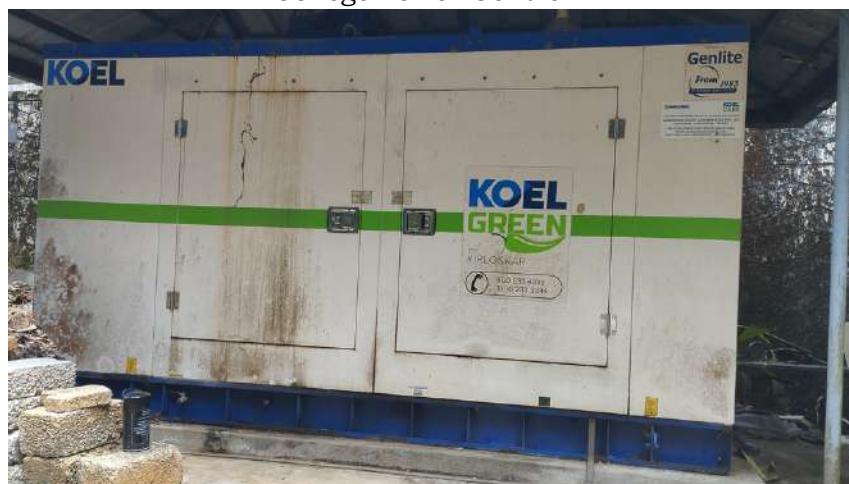
Standby Power Generator 125 kVA
